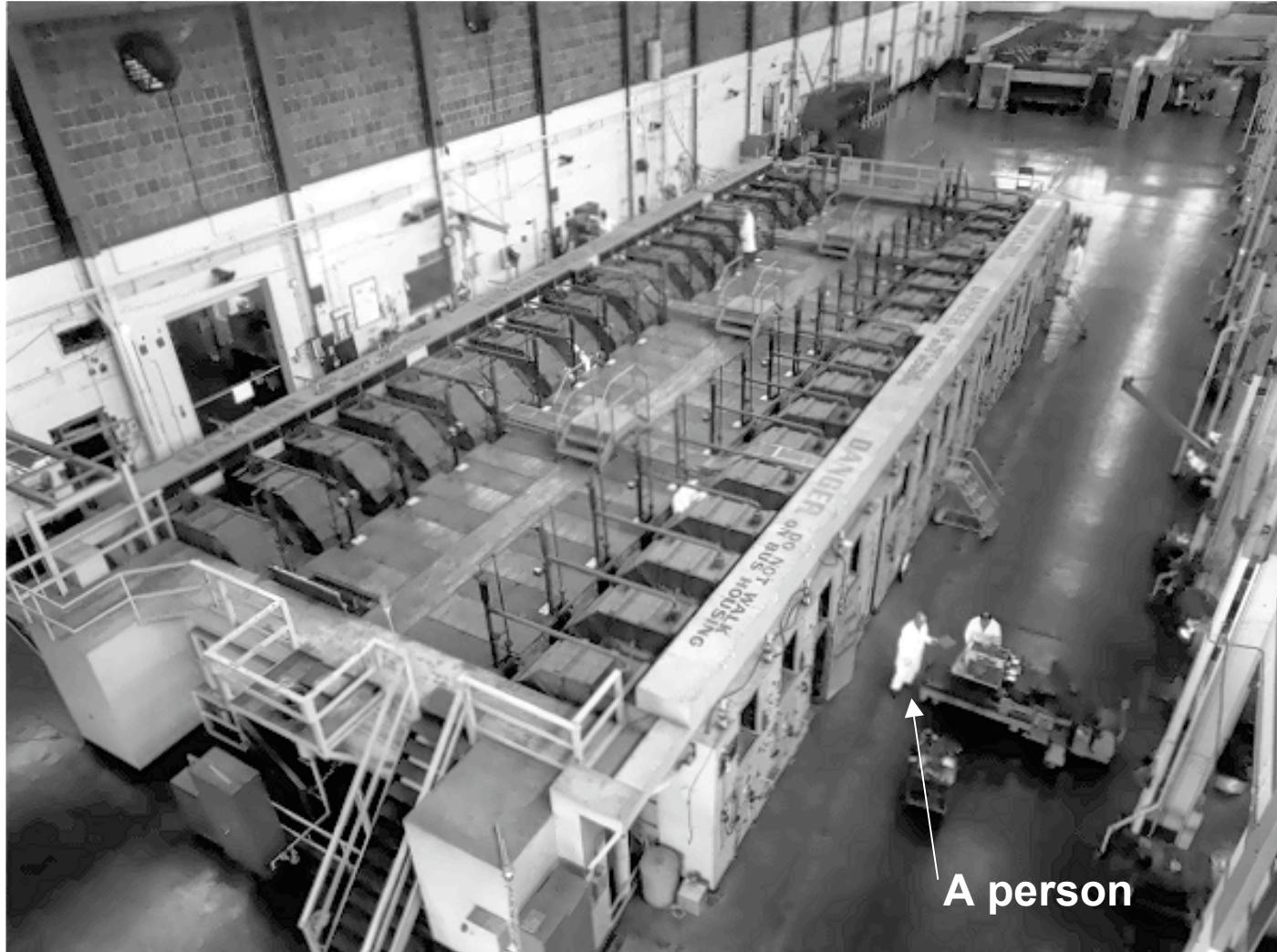
A bank of 32 Calutrons (of 1152 built) for preparative MS of isotopes at Oak Ridge built circa 1945
